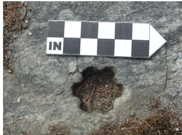
less technical terms, the rifled star holes are the result of the drill bit chattering in the hole. The chattering was most likely the result of several factors including the vibrations caused by the drilling machine, a dulling bit, metal fatigue in the drill rod, and the rotational speed of drill.
